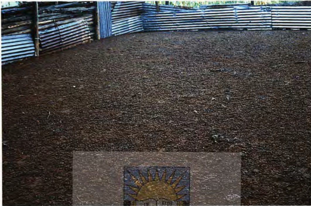
Plate 4.4. The walls of a corrugated iron kraal are usually made of old roof sheets but some farmers purchase new sheets when building a kraal.
