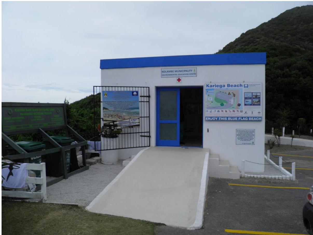
Figure 2: Example of the environmental information centre in Kariega
