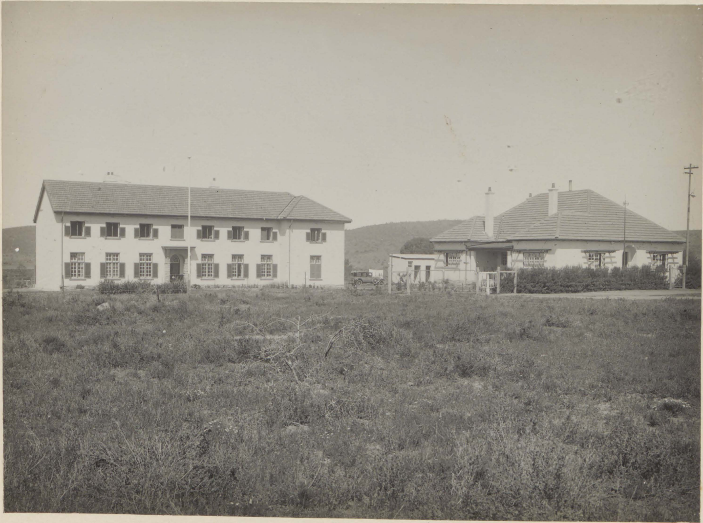
Presbyterian Hostel. & Warden's Residence.
