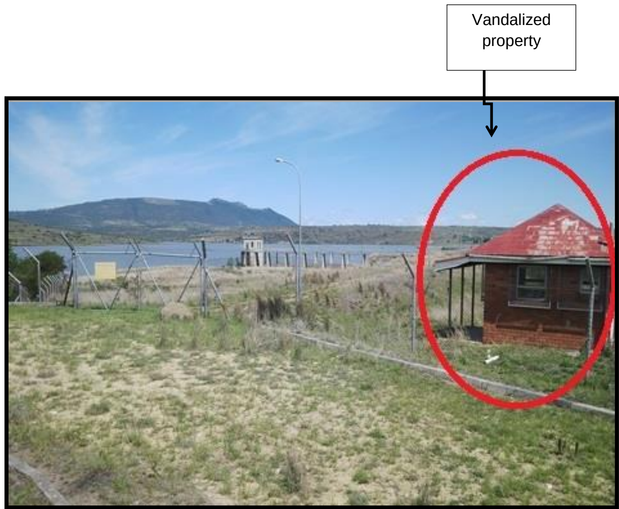
Figure 4.6: Vandalized property at Binfield, Alice, Eastern Cape, South Africa (2014)
