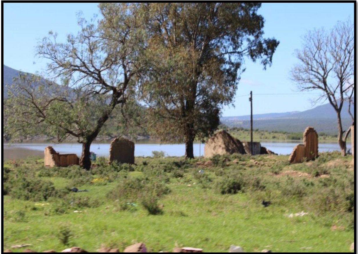
Figure 4.3: Demolished houses (10m) next to Kat River Reservoir, Seymour, Eastern Cape, South Africa (2014)
