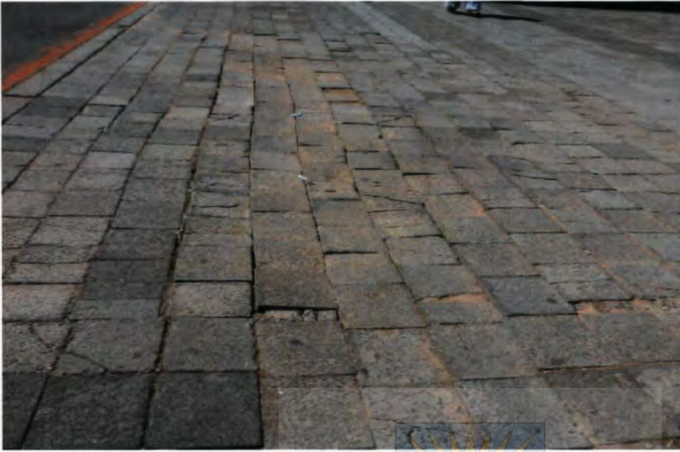
PLATE NO. 5: Pavements (East London CBD)
