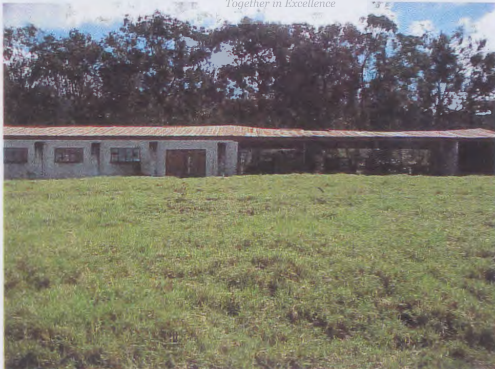
Picture 2: Tools and machinery shed
