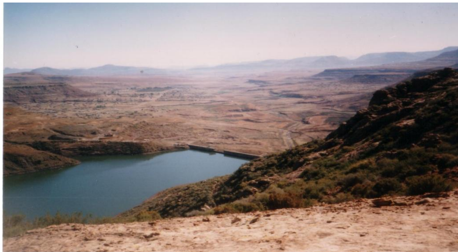
Figure 5.28 The Halahlahatsi dam, situated just south of Magwiji village (September, 2007)
