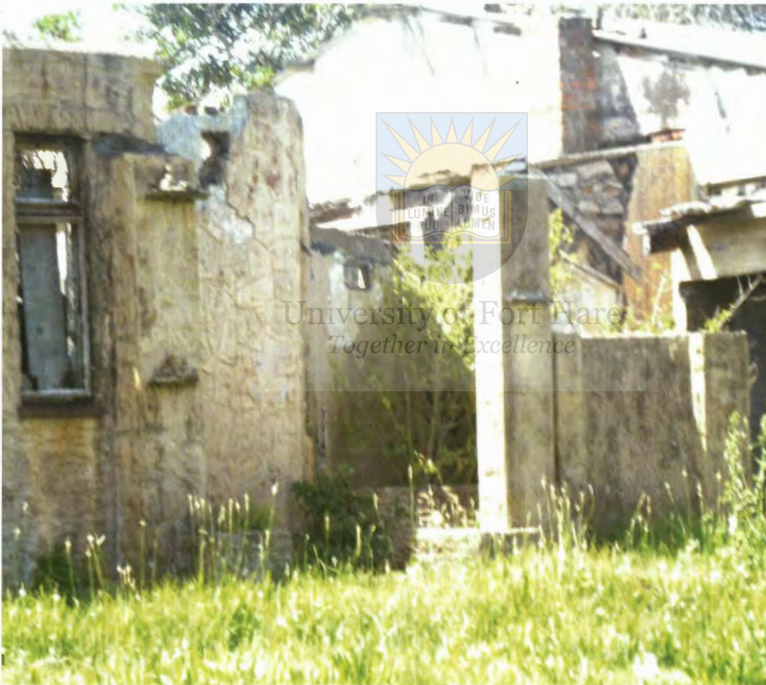
Picture 3: A dilapidated house in Cocobana
