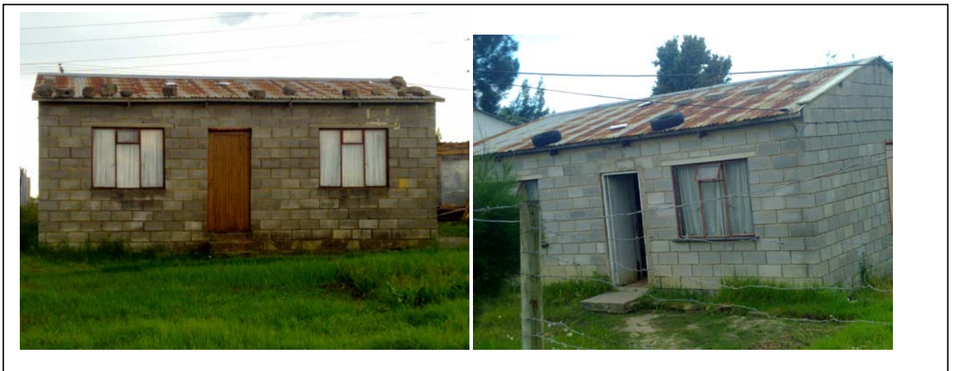
Picture 6. (The roofs are not rigid that they are supported by heavy stones and old tyres)
