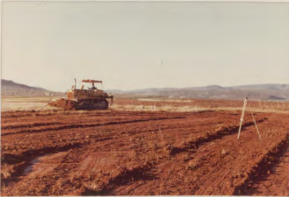
Removing grass and topsoil from pond site, Tyefu Integrated Unit
