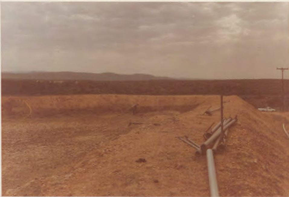
Dam walls complete, tenant spreading lucerne hay lining. Irrigation pipes ready to wet lining
