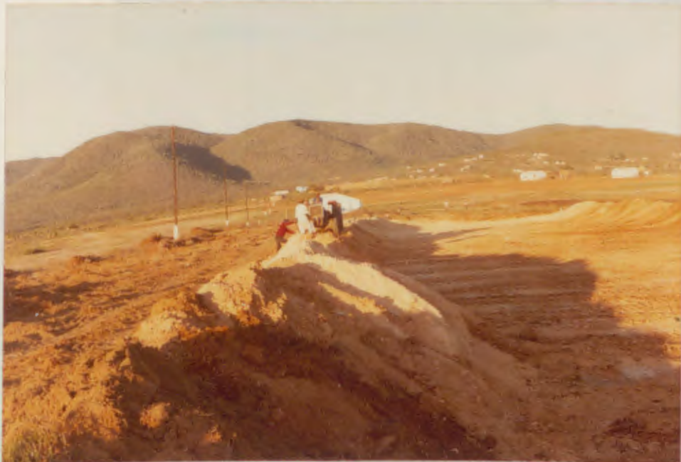
Compaction of second layer on dam wall
