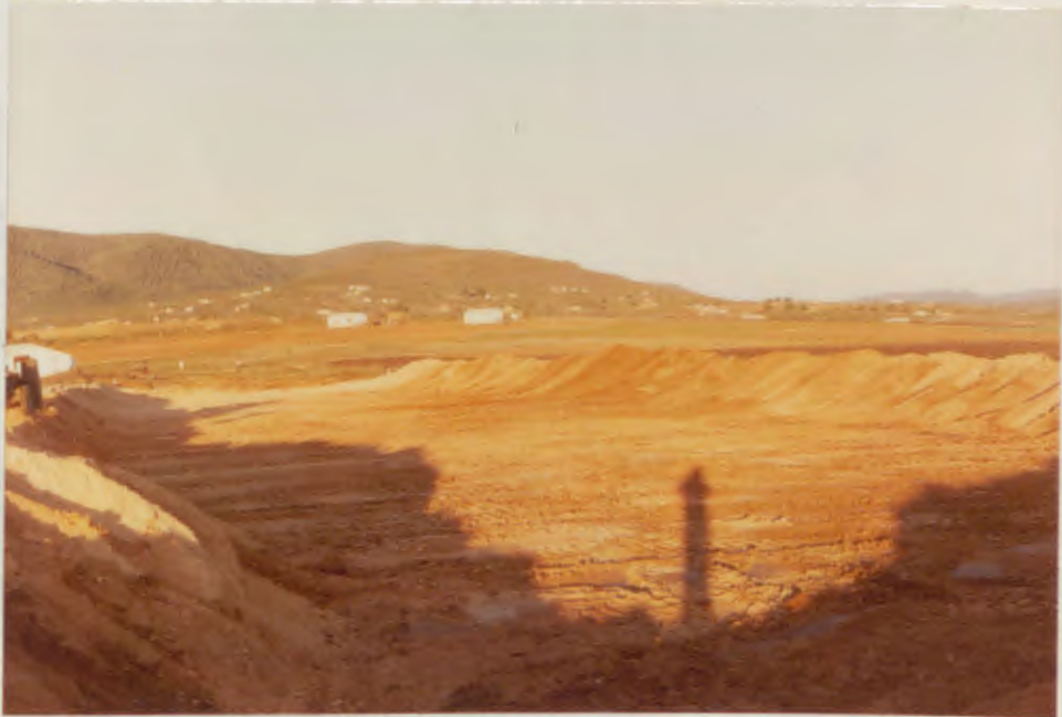
Pond base level with no more soil to be excavated
