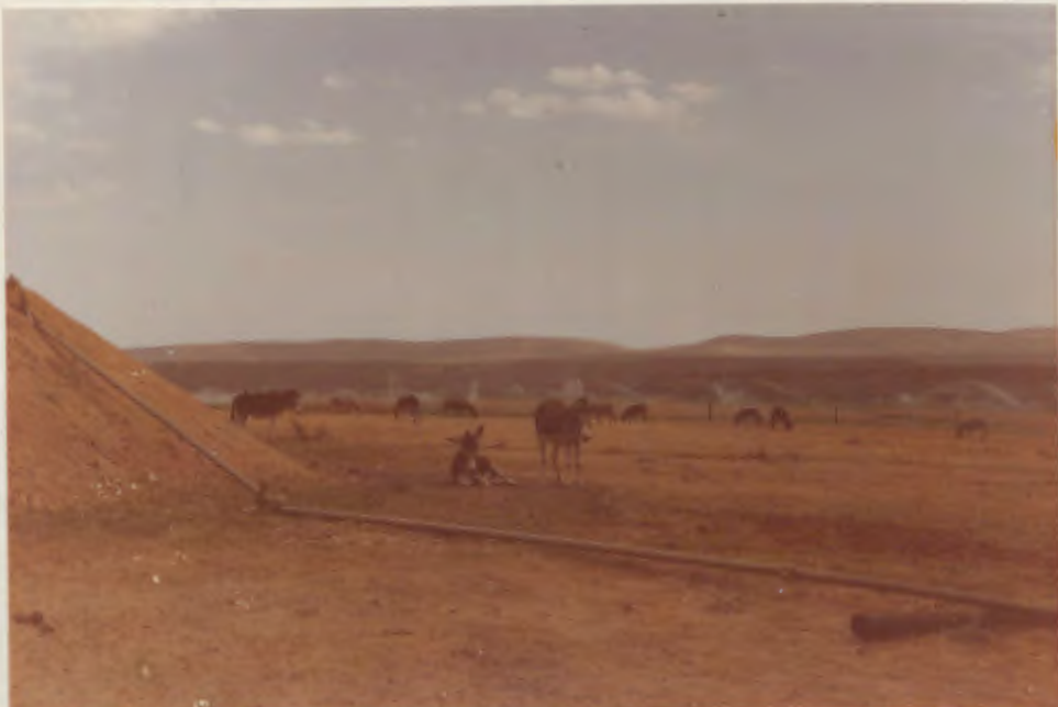
Donkeys were used to assist puddling pond floor
