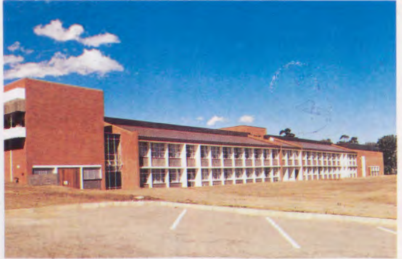
The west and south sides of the new block.
