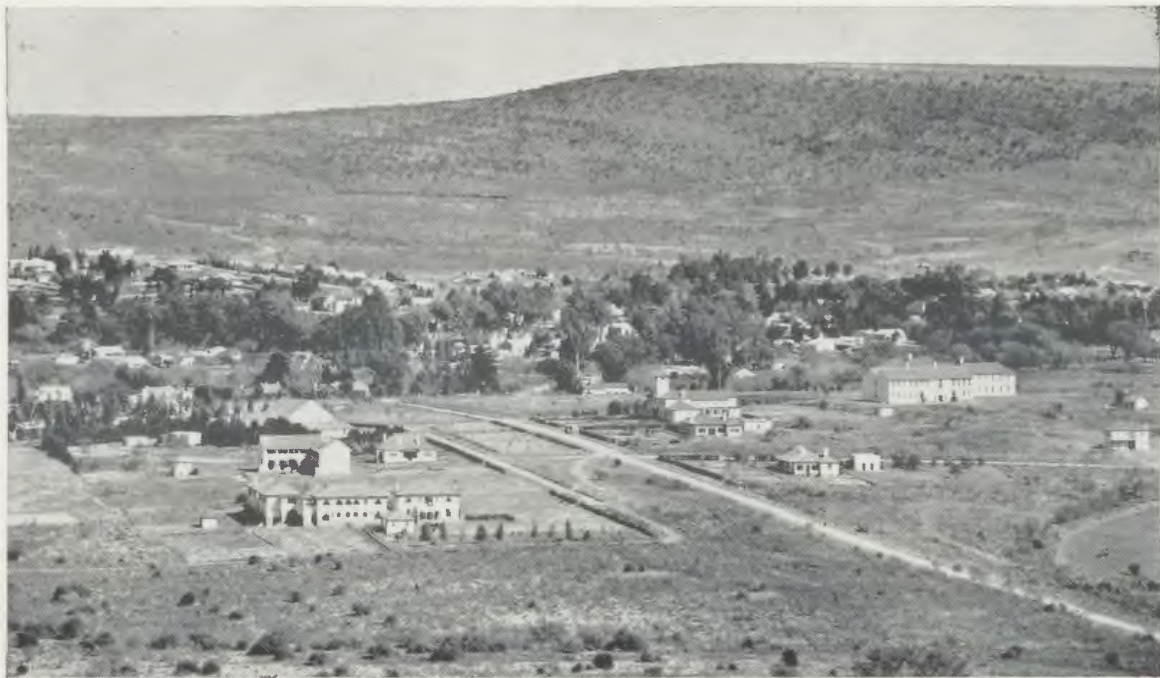
FORT HARE GENERAL VIEW.
