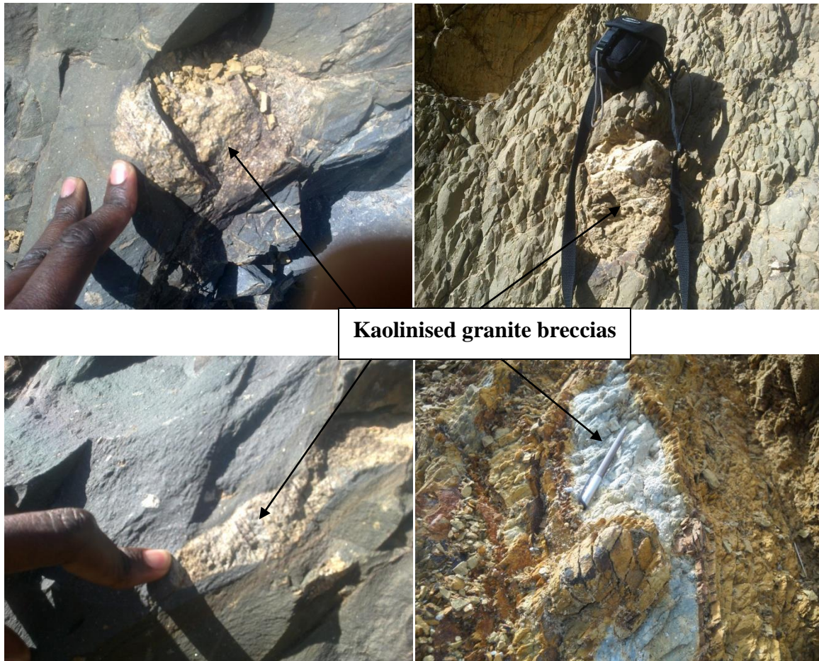
Figure 6- 17: a, b, c, and d; Fractured granite breccias in advanced stage of weathering, the kaolinisation start to develop in the granite breccias (well seen in Figure 6.17 d)
