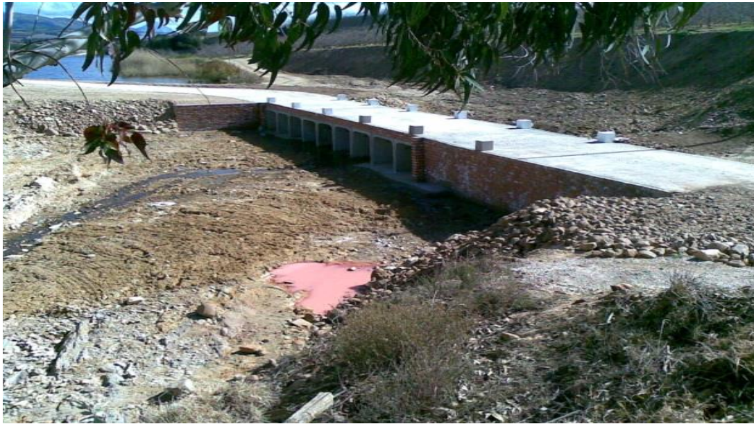
Figure 3.4 Photograph showing the bridge built in 2007 by Department of Rural Development and Agrarian Reform Source: DRDAR, 2013
