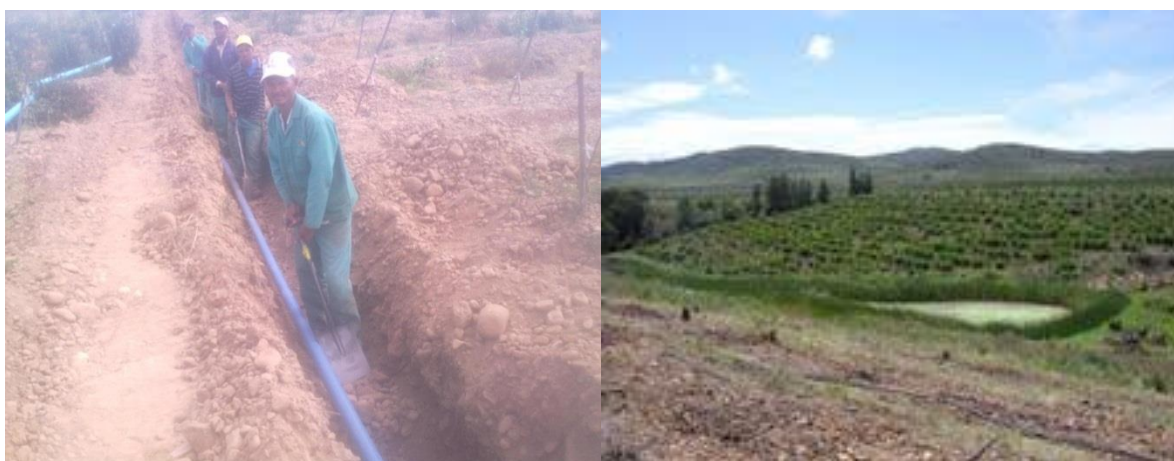
Figure 3.7 Photograph showing trenches for new irrigation system and the dam, built 2011/12 and 2010/11 respectively (Source: DRDAR, 2013)
