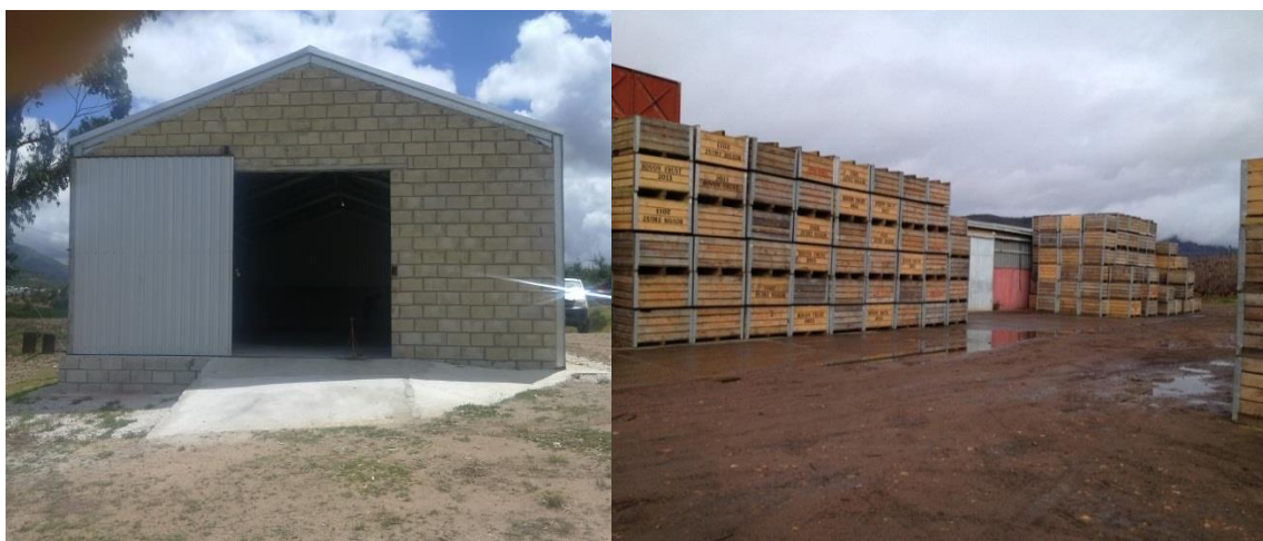
Figure 3.8 Photograph showing new storage shed built on 2013 and harvesting bins bought on 2011
