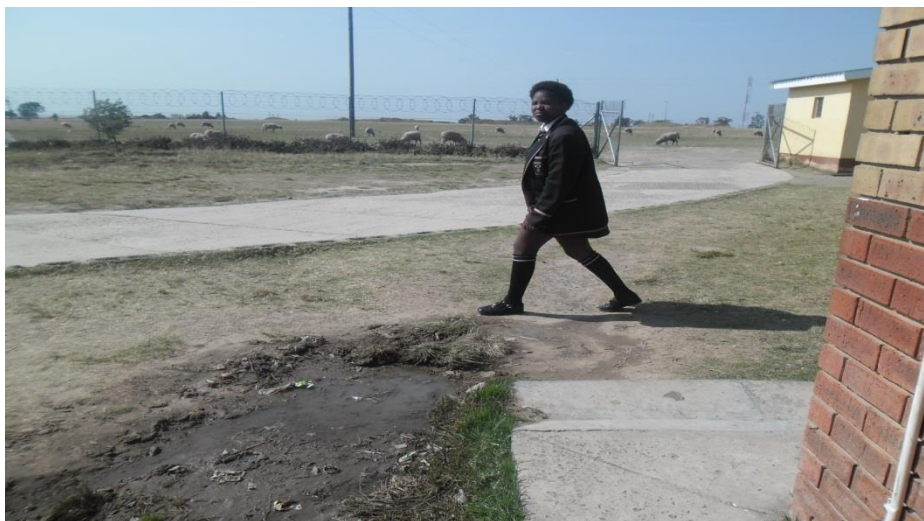
Figure 4.1: Gates wide opened for free entry and fence of wire mesh around the school yard
