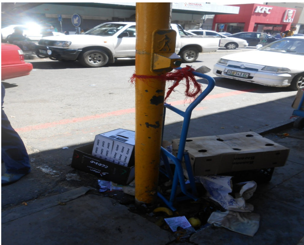
PLATE NO. 8: Traffic signal (East London CBD)
