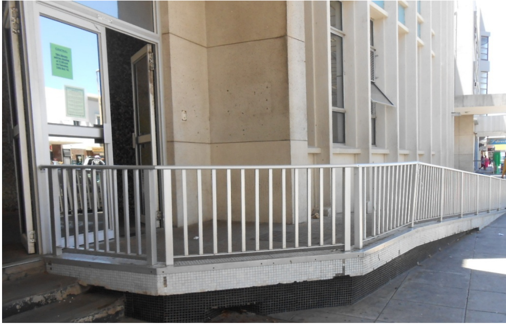
PLATE NO. 13: Ramp and door (East London CBD Library)
