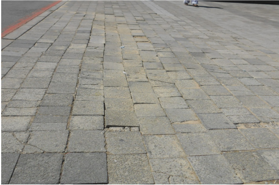
PLATE NO. 5: Pavements (East London CBD)
