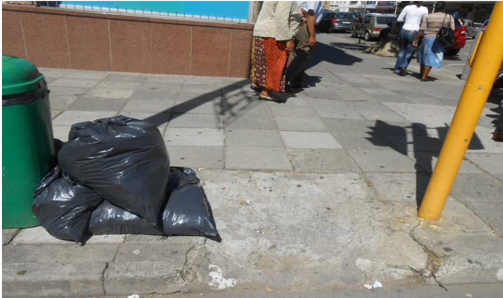
PLATE NO. 7: Kerbs at a traffic signal (East London CBD)
