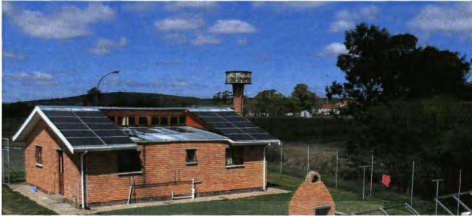
Plate 3.1: Photo of the passive solar house
