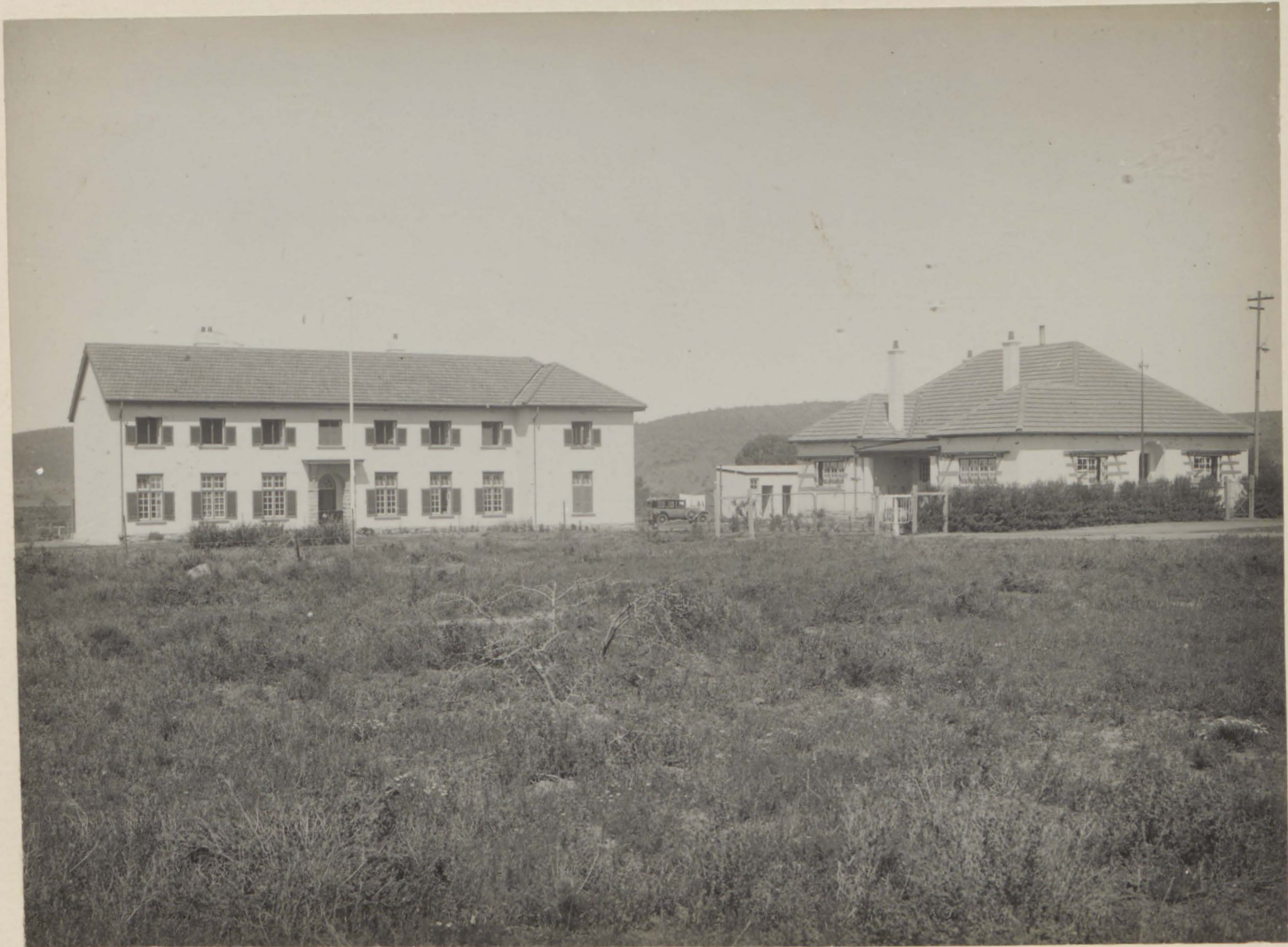
Presbyterian Hostel. & Warden's Residence.
