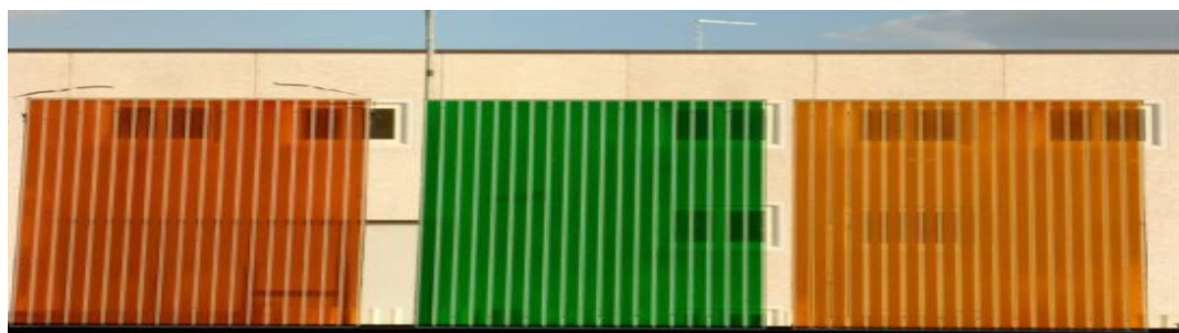
Figure 10: The modules or panels of solar cells built from three different types of dye-sensitized solar cell.
