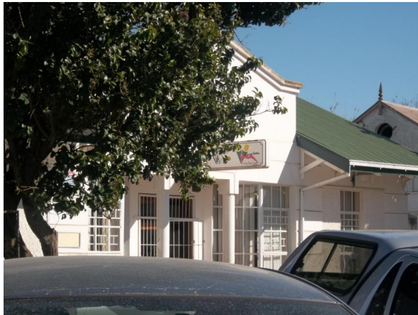
Photograph 4.1: Africare offices in Alice, Eastern Cape
