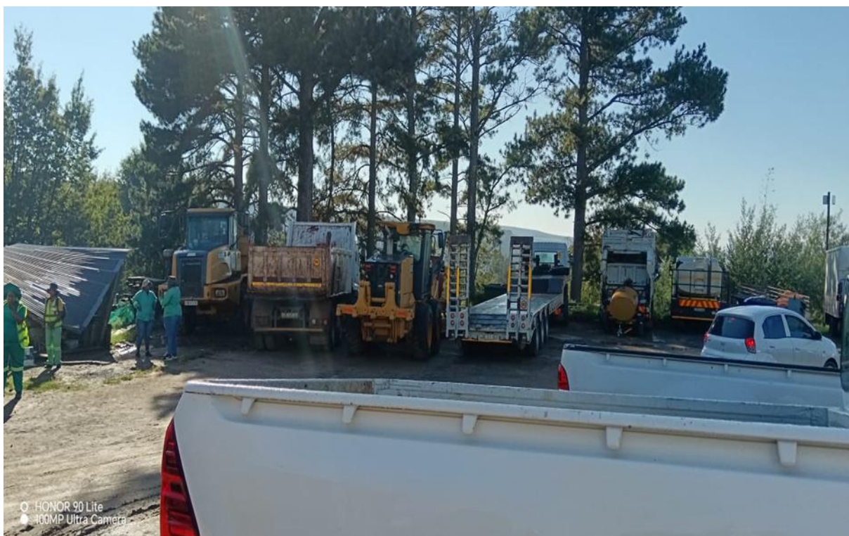
Figure 1: ELM equipment for road maintenance
