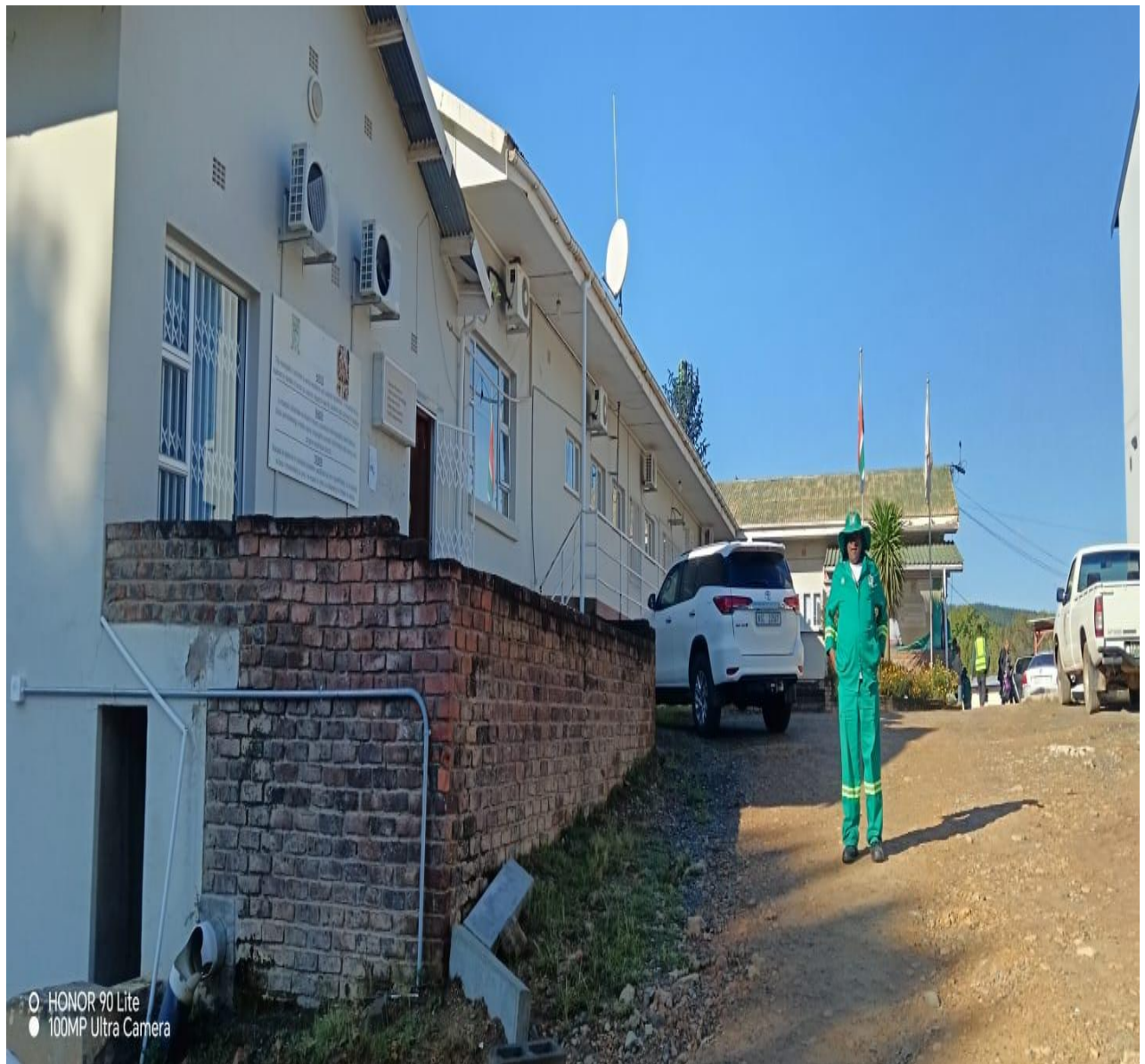
Figure 8: Elundini Local Municipality Main Building
